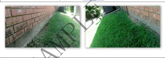
Downspouts dispensing water too close to the structure. It's recommended that the downspout be extended 18"-30" from the structure or an adequate alternative method applied. [Front, towards the center of the structure.(When facing the front)] - "§535.228 (b)(1)(C)"
